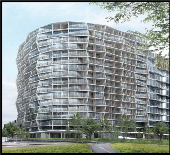
Figure 1: The CAD model of the Nishi Apartment building in New Acton (Molonglo Group, 2011).
