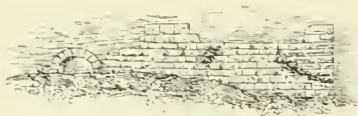
The N Wall W Building
